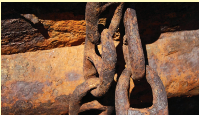
Fig 3.6. Rusting of iron
