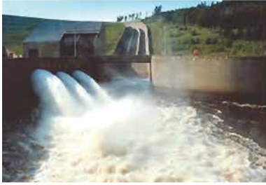
Hydro electric power station
