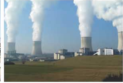
Thermal power station
