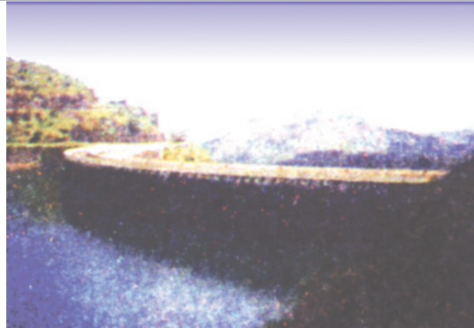
Arch Dam - Idukki
